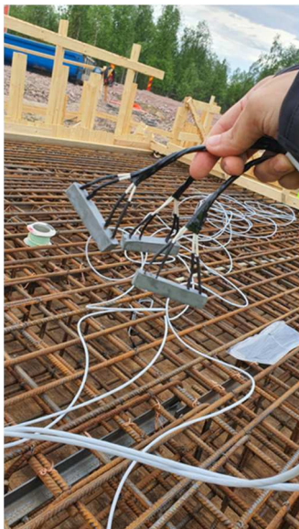
Figure 4-23 SmartCem sensors ready to be installed (left) and after installation of SmartCem sensors at the studied locations (right)
